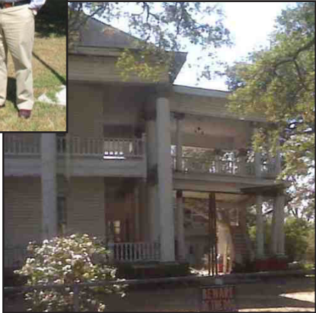
A view of the 1901 Carter House's failing porte cochere.
