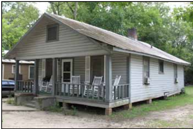
This house at 1004 Lester Street is one of the 2010 Operation C.A.R.E. Houses that need your help!
