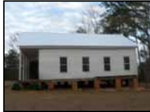
Roof Work Completed January 2011
