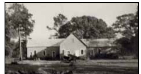
At Right: Old Metcalfe School (lost)
